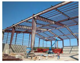
Concrete push walls and sturdy construction are needed at solid waste transfer stations. High ceilings allow for the opening of compactor trucks and dump beds within the containment of the building. This new construction was at the Tazewell Transfer Station, that opened in January 2008.
